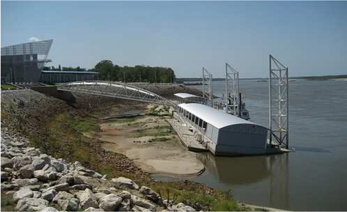
The dock at Tunica is on the ground and tilting due to the low water
